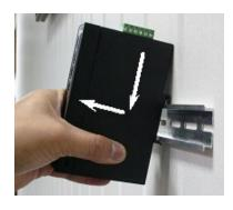
**Step 2:** Lightly press the button of DIN-Rail for remove it from the track.
