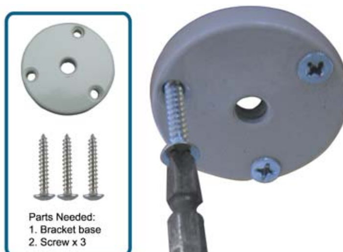
Figure 2: Screw the base to the ceiling
